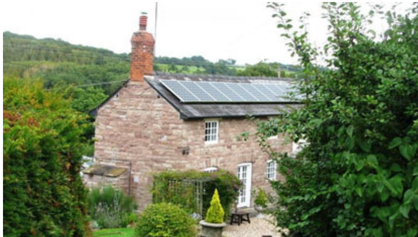
Keel House Panels on the roof
